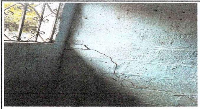
FOTO 3: SE OBSERVA GRIETAS Y FISURAS EN LAS PAREDES.
