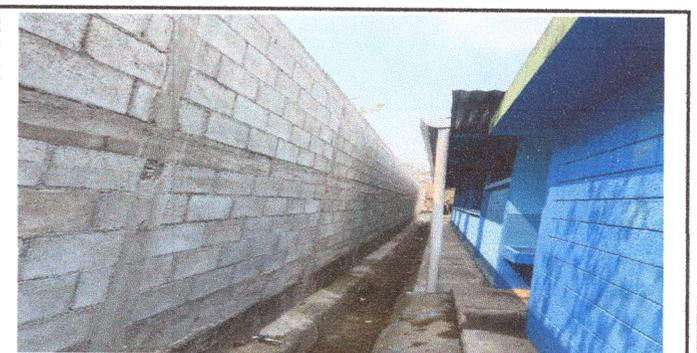
Foto 6: REEMPLAZO DE LA MALLA POR MURO DE BLOCK CON COLUMNAS Y SOLERAS Y ZAPARAS A UNA ALTURA DE 2.40MT DEL NIVEL DEL PISO
