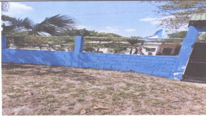
3. MURO PERIMETRAL, 70 ML
