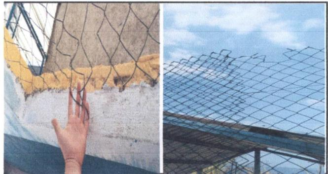
**Foto 6: SUSTITUCION DE MALLA EN MAL ESTADO PATIO PRINCIPAL**
