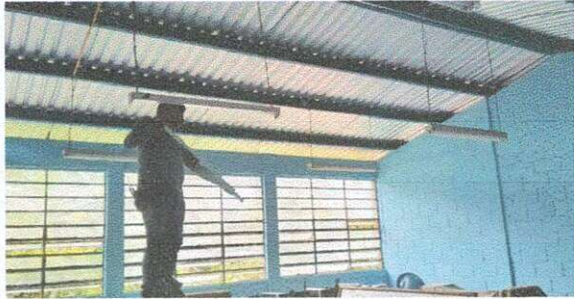
Foto 9: Instalando tubos Led
