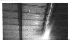
Foto 11: CAPOTE Y LAMINAS EN MALAS CONDICIONES, LAS LAMINAS PRESENTAN OXIDO
