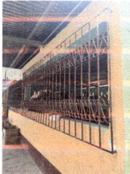
Foto 7: ESTRUCTURA EN MAL ESTADO, LAMINAS CON OXIDO, MALOS TRASLAPES, RAJADURAS, BALCONES DAÑADOS
