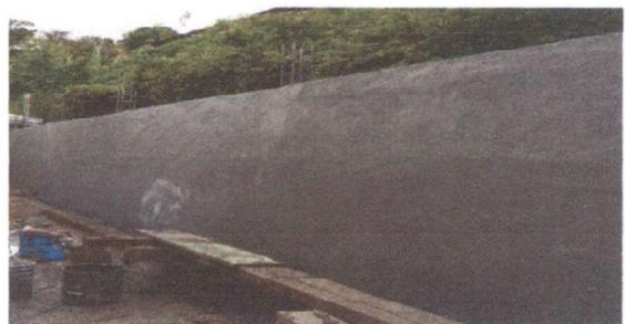
Foto 10: PINTURA EN MURO PERIMETRAL
