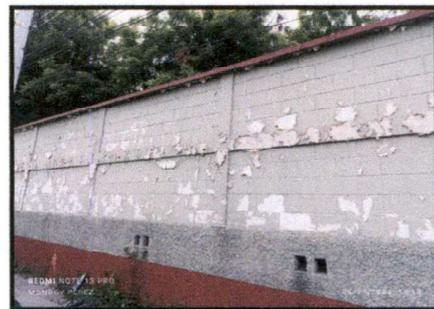
Foto 6: REZANE DEL MURO PERIMETRAL EXTERIOR.
