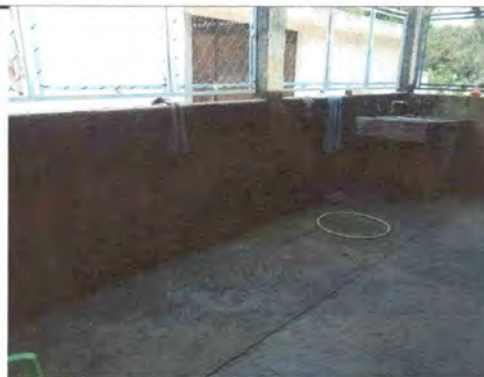
Foto 4: Replacement of pile by pile made of cement.
