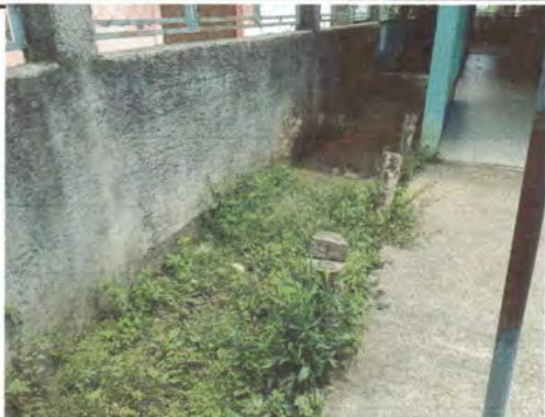
Foto 1: Continuation of patio roof.
