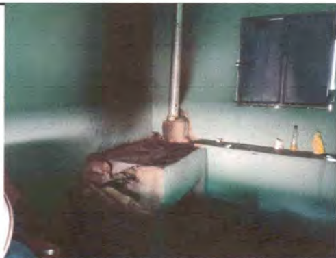
Foto 3: Repair of polletón and replacement of plate.
