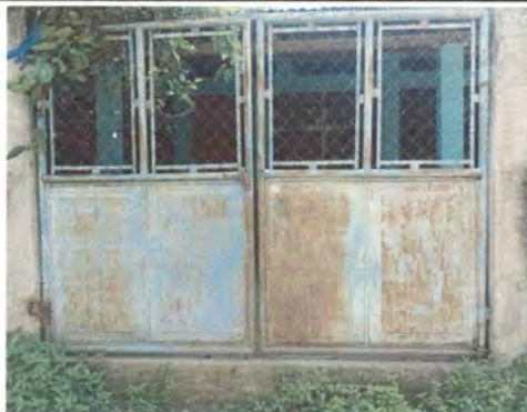
Foto 2: Maintenance of gate (brushed, sanded, and painted).
