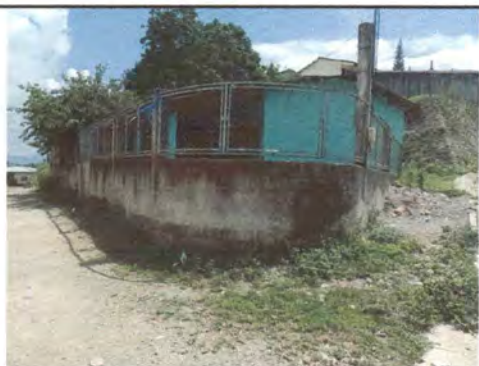
Foto 5: Painting of exterior and interior walls of establishment.
