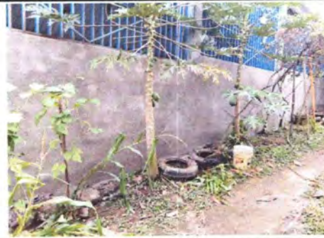
Repello de pared exterior
