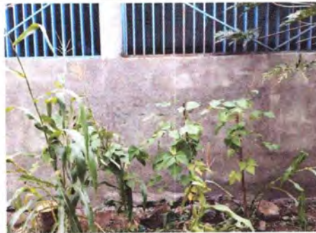
Repello de pared exterior
