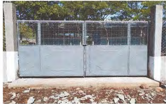
Porton Ingreso Principal
