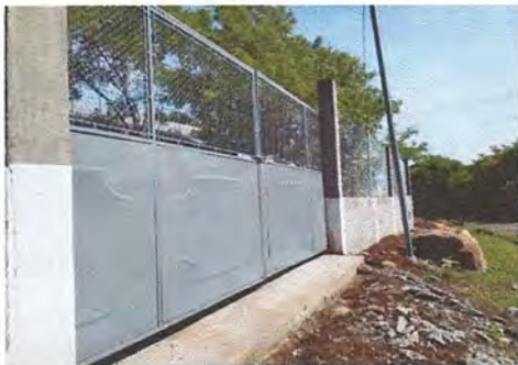
Porton Ingreso Principal
