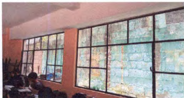
Foto 1: colocar balcones no. 5
