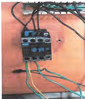
REINSTALANDO CEELECTOR ELECTRICO
